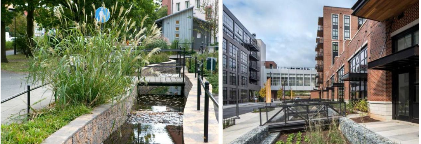
Figure 12-9. 2. Alternative Stormwater Detention Facilities
