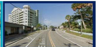
Existing Segment D
